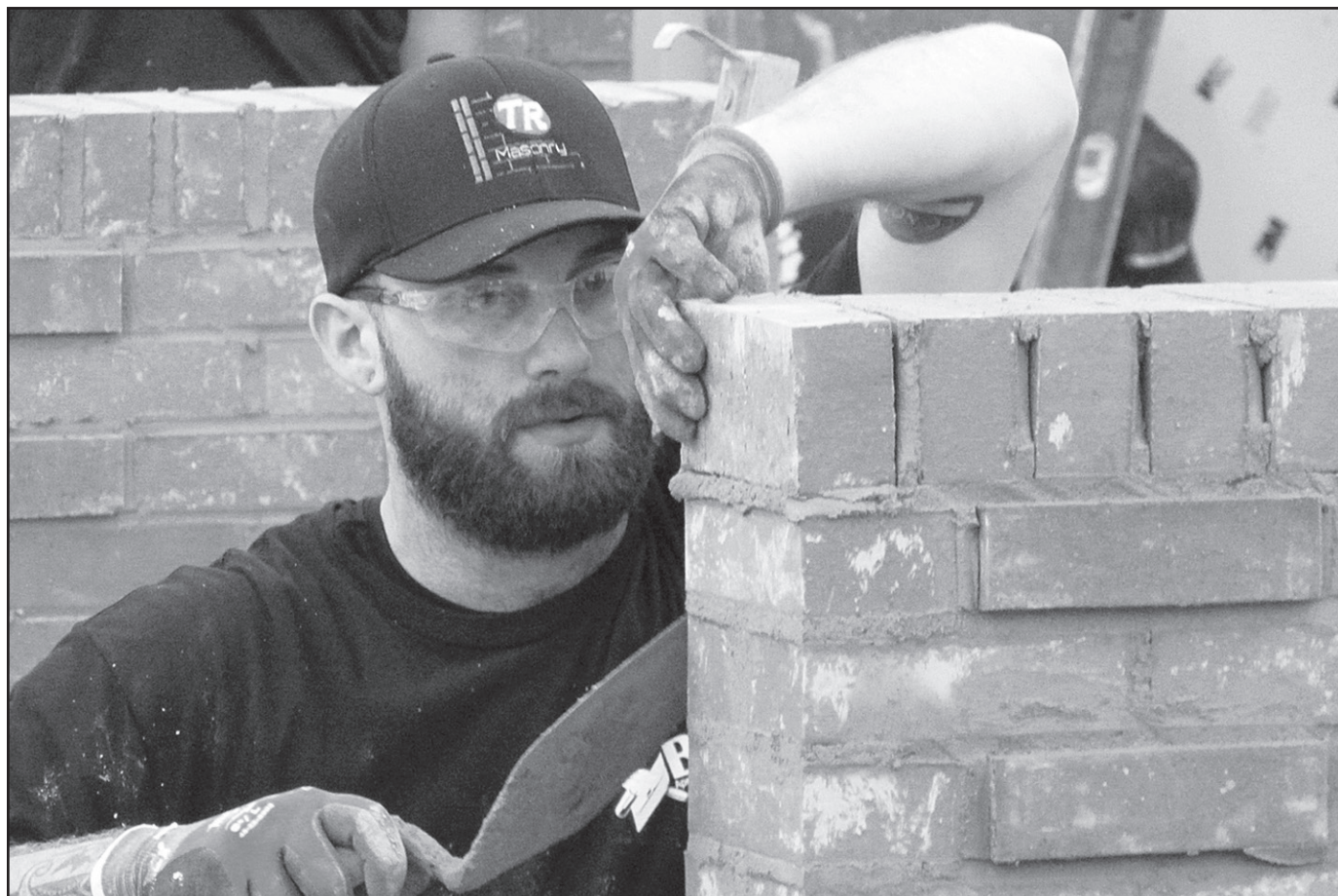
Photo above: Keanan Carlson, second year apprentice, laying the final course of his project, a rowlock course.
