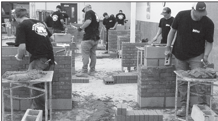
Photo above: The Bricklayers Local 1 training center is located in New Hope.
